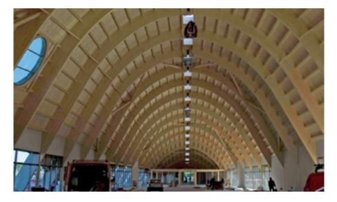
Architektur, Eckernförde, is based on an idea of Bauplan Nord GmbH & Co. KG, Flensburg. 25 plank trusses span the 125 metre long, 25 metre wide and up to 15 metre high vaulted structure. Window panes in the front area of the hall provide for sufficient daylight illumination. The entrance to the "playing whale" is located in its tail fin. And through the giant jaws little and big visitors can access the outdoor area of the playground.
