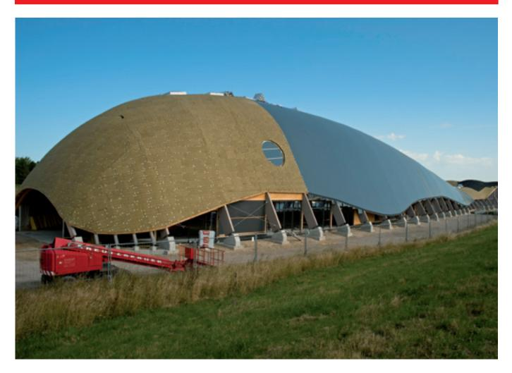
The exposed location of the building was another challenge as strong winds were more or less constantly blowing during the installation of the outer covering of the whale. The wooden supporting structure was manufactured by Gebrüder Schütt KG from the town of Landscheide, and the remaining works on the outer roof construction were carried out by the roofing company Karsten Poppner from the town of Kappeln.
