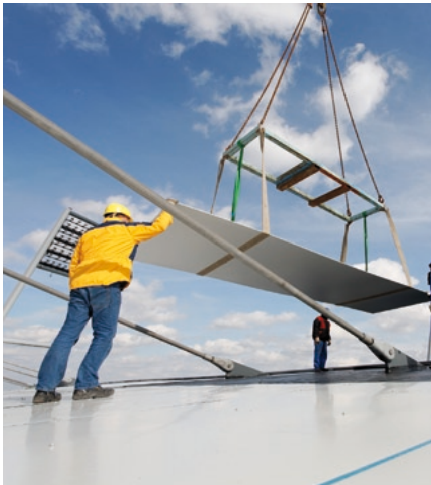
▲ Installing plain sheet metal for an even roof area
