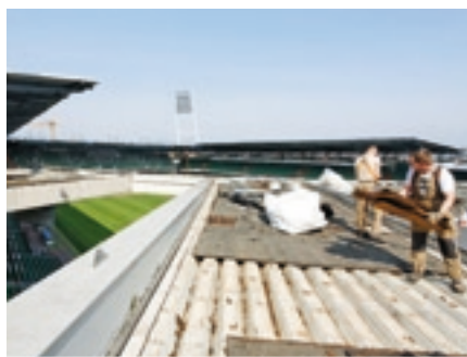
▲ Dismantling the old roof build-up
