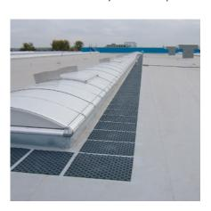
for load distribution. Movement of the maintenance walkway tiles even at increased wind loads is prevented by hot air welding the tiles to the EVALASTIC® waterproofing membranes. The visible delineation between waterproofing membrane and maintenance walkway tiles has the advantage of clearly marking the roof areas (inspection and maintenance walkways) people can safely walk on.
