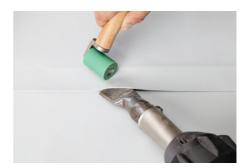
The plastified lap areas will be fused by applying moderate pressure with a silicone pressure roller, following parallel to the opening of the nozzle. Due to the backwards movement, the nozzle always blows against already seal welded areas of the seam.
