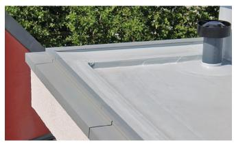
Note: With the flashing against the roof sealing being set back by 120 mm, rainwater in this area will drain off over the front surface of the profile!
